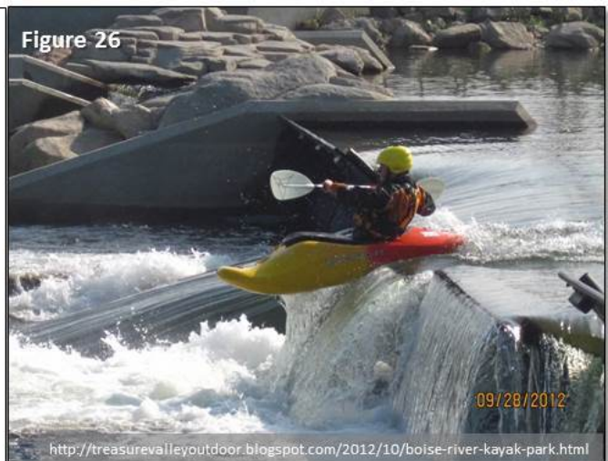
Figure 26: Boise River Whitewater Park wave. Sections of the dam can be raised or lowered incrementally to shape waves, impound water for irrigation purposes, or increase flow and sediment passage.
